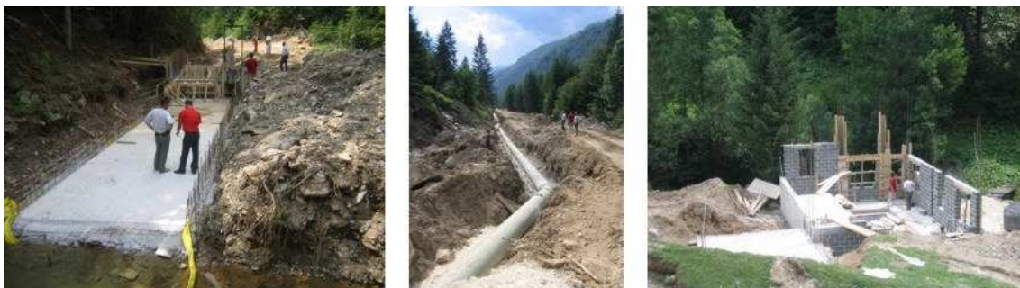
Figure 2.5. SHP plant in construction on Prusacka River at Vranica Mountain - water intake, penstock, powerhouse
