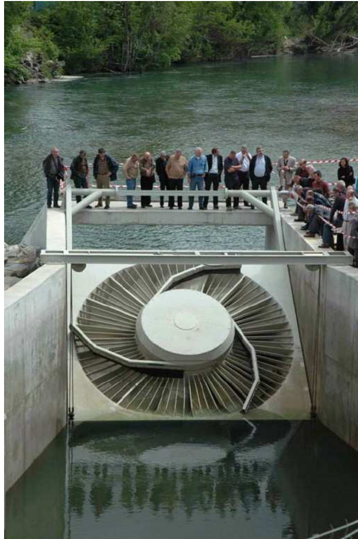
Figure 23 – VLH in working position during the visit of 50 power plant owners
