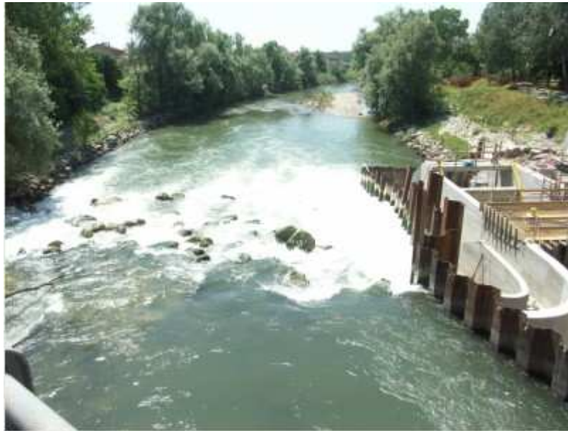
Figure 7 – Power plant under construction on site n.2
