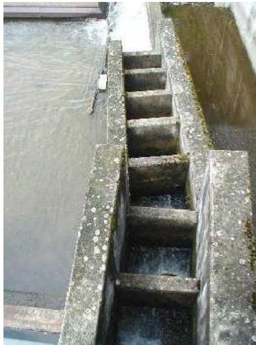
Figure 25 – Fish-ladder as series of pools one above the other, with water overflowing from the higher ones to the lower ones
